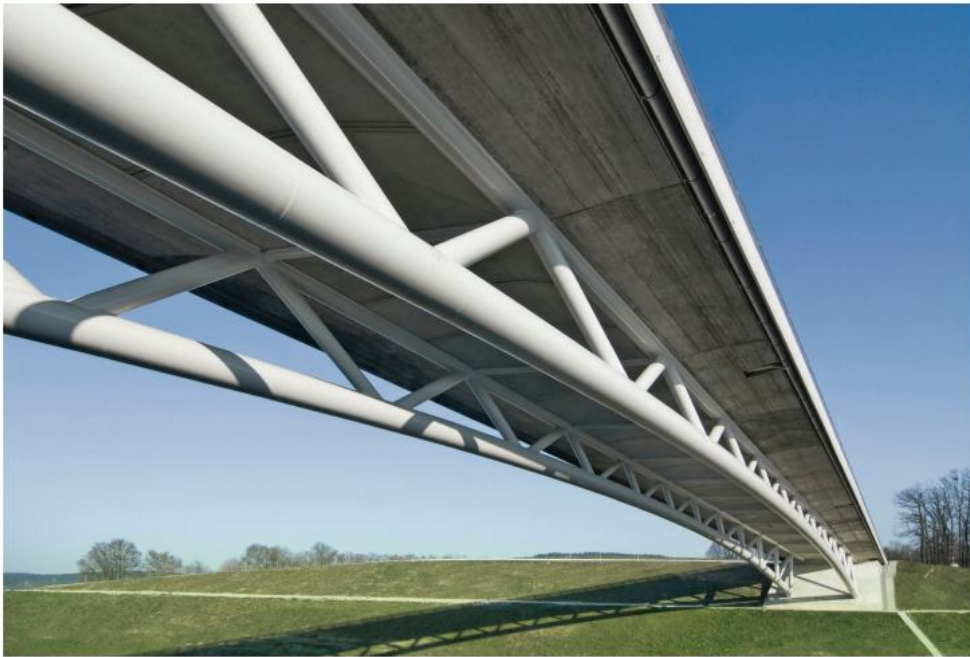
Composite bridge with integral abutments (Munich), Germany
