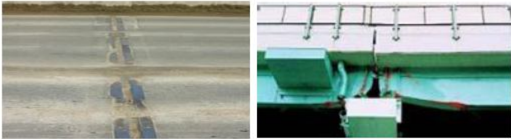
damaged expansion joint bridge
