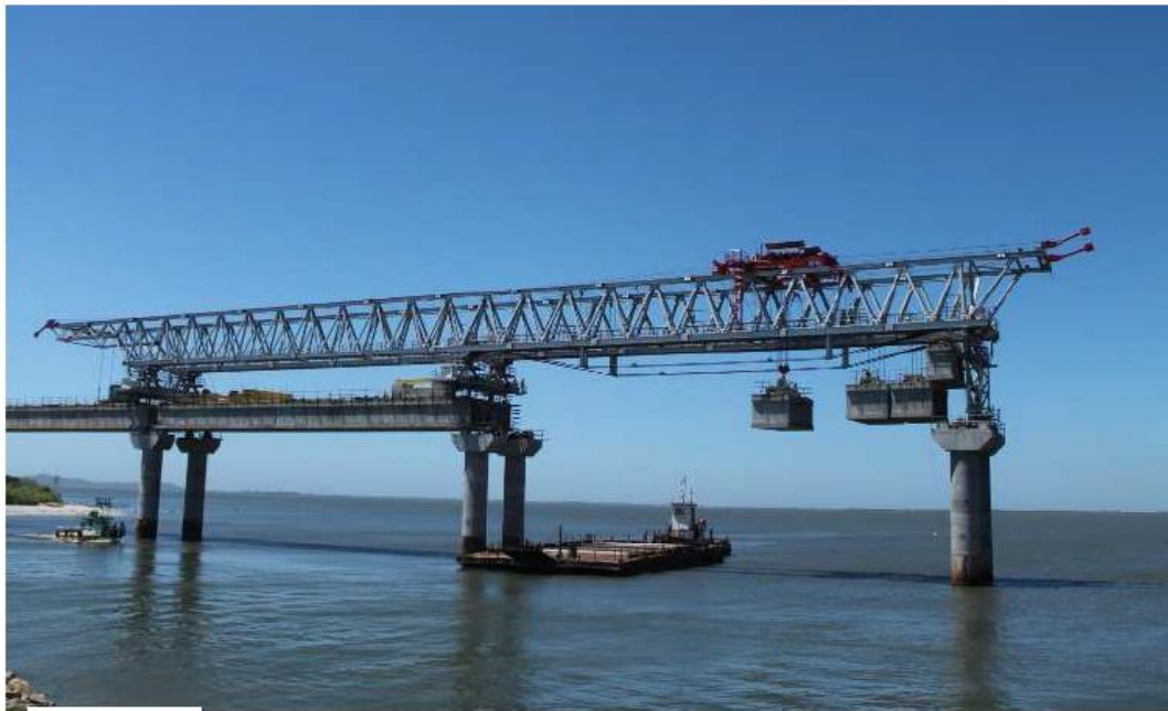
Launching gantry for span by span precast segmental construction (50 m spans)
