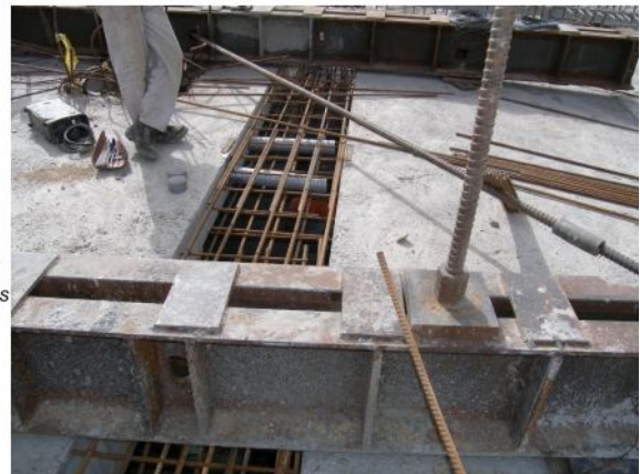
Typical erection equipment for closure joints in cantilever bridges
