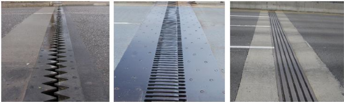
damaged expansion joint bridge
