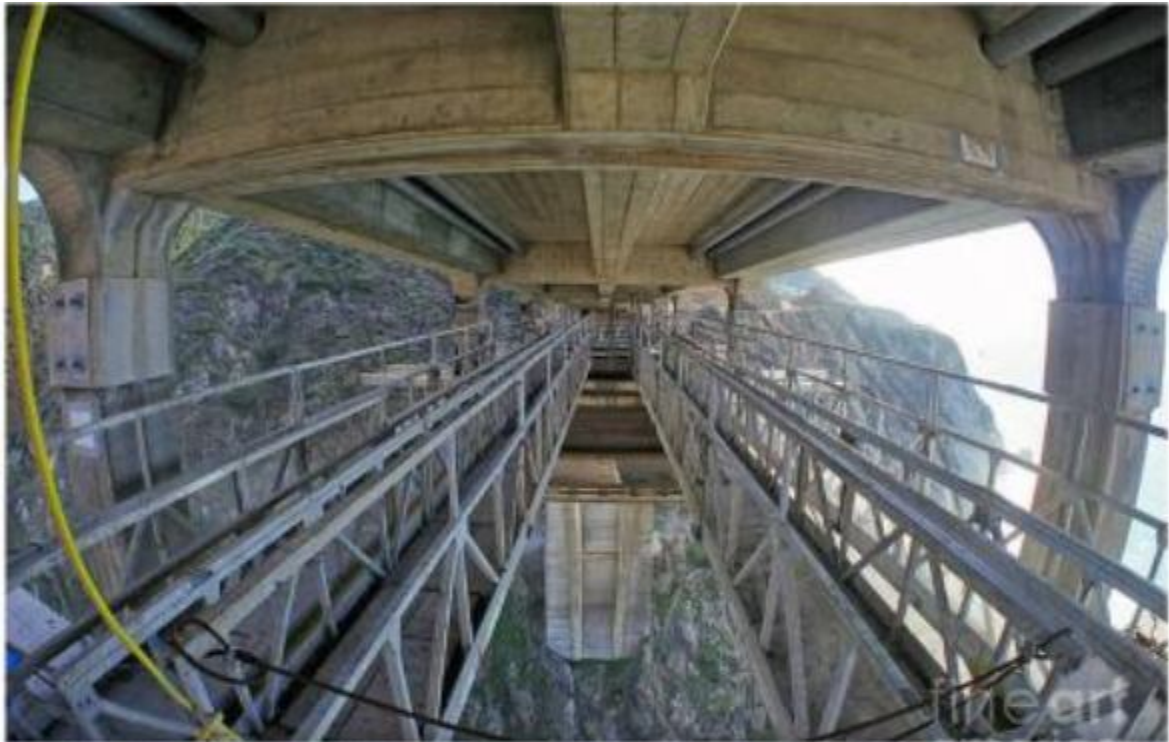
Looking South on the temporary deck under the roadway of Bixby Creek Bridge during the seismic retrofitting project.
