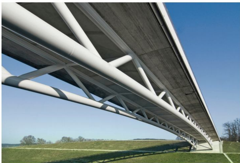
Composite bridge with integral abutments (Munich), Germany
