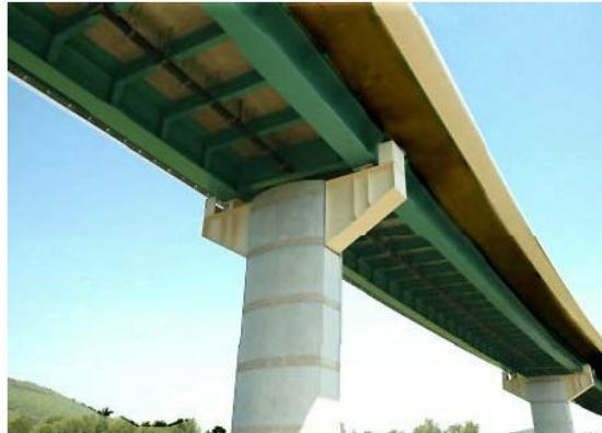
Two girder composite deck
