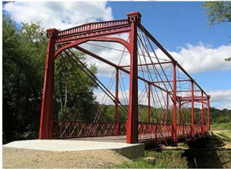
Quadrangular Truss.
